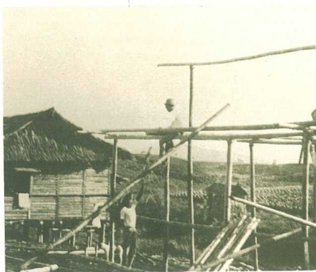
Early housing settlement (Camp I, December, 1928) for plantation workers who were mostly migrants from neighboring islands.
