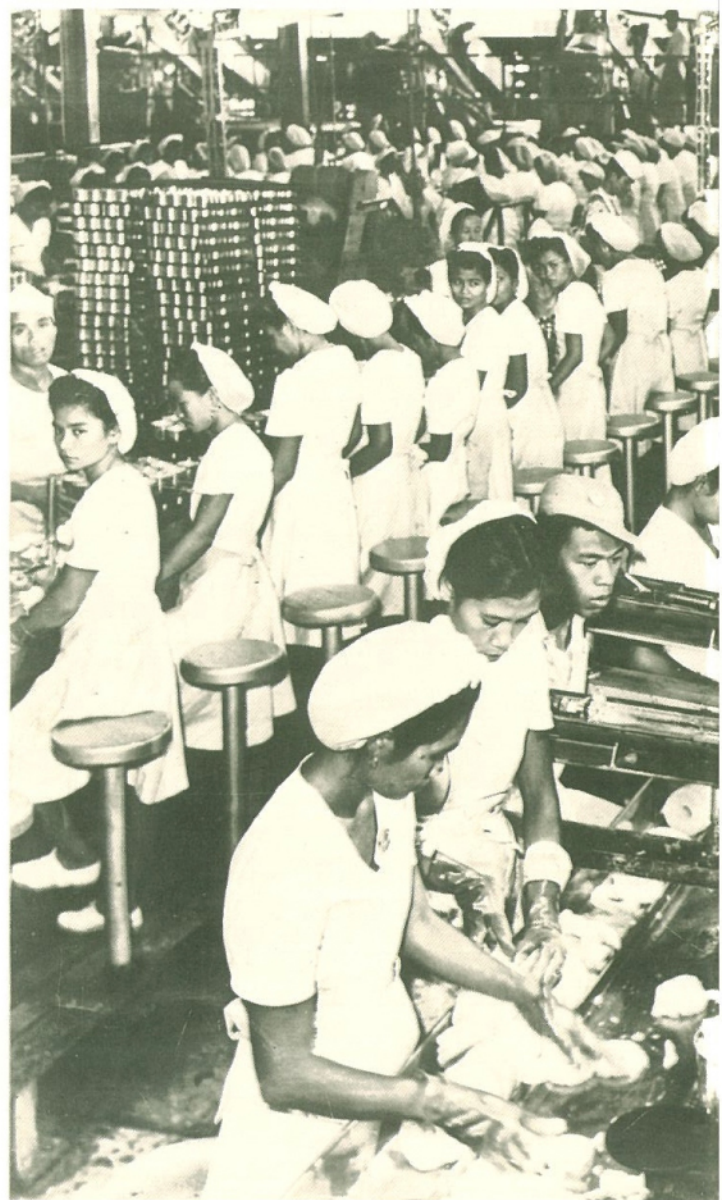
The rehabilitated cannery after the war. Reconstruction work started from scratch.
