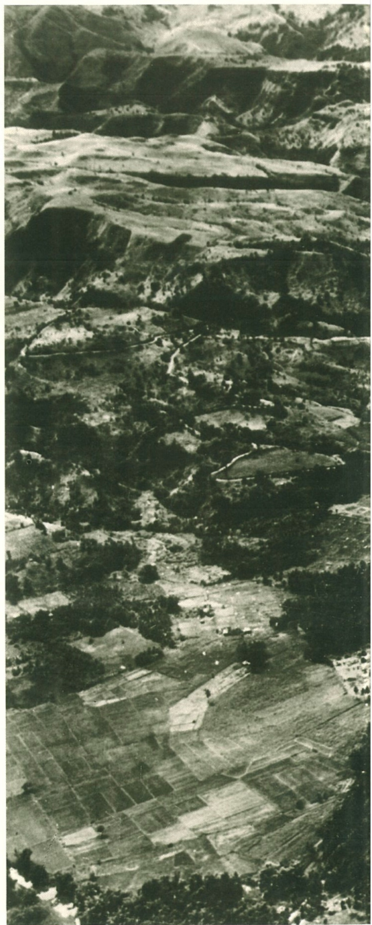
Aerial view of Bugo cannery in Cagayan de Oro taken in November, 1930.
