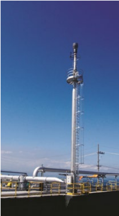
DMPL's waste-to-energy facility in the cannery
