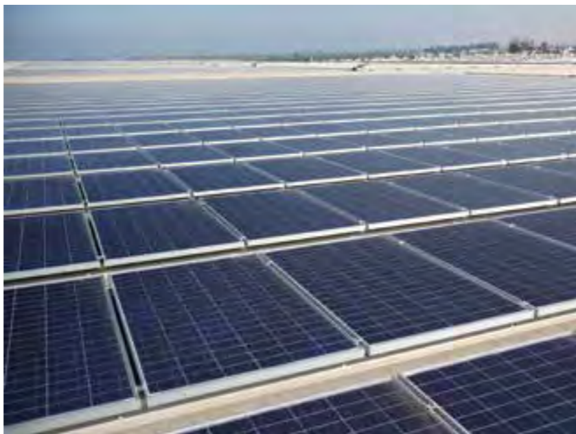
Solar panels in Hanford facility in California
