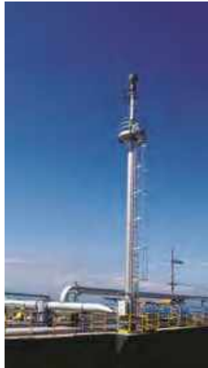
DMPL's waste-to-energy facility in the cannery
