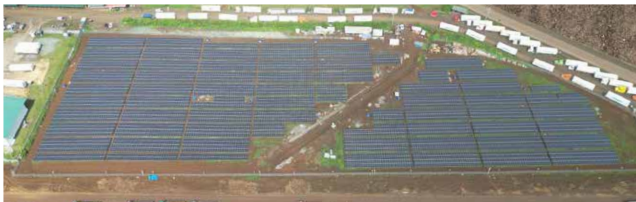
Solar energy facility located in Manolo Fortich, Bukidnon, close to manufacturing facilities
